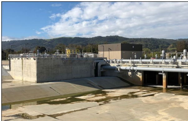
DSRSD basins stand ready to receive and store secondary effluent supply prior to the ballasted flocculation process.
