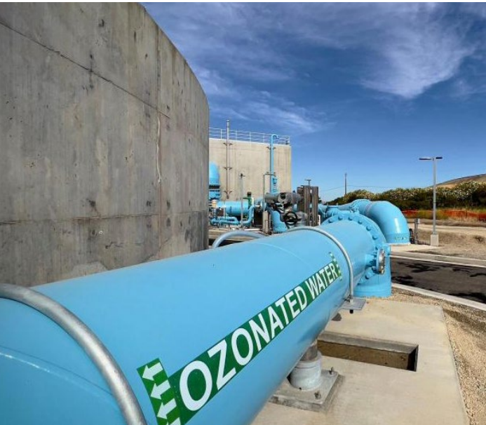
Zone 7’s Patterson Pass Water Treatment Plant uses ozone as its main disinfectant for water from the State Water Project.
