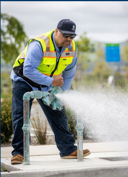
A DSRSD employee opens a test cock on a backflow prevention device to verify that it is receiving water flow.
