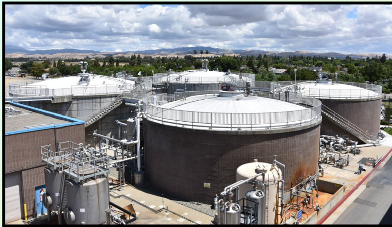
Anaerobic Digesters
