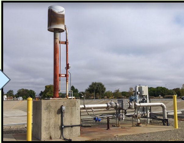
Waste Gas Burner (Biogas Flare)
