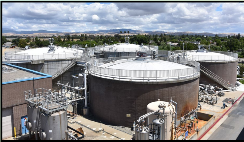
Anaerobic Digesters
