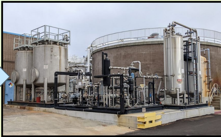
Biogas Conditioning System
