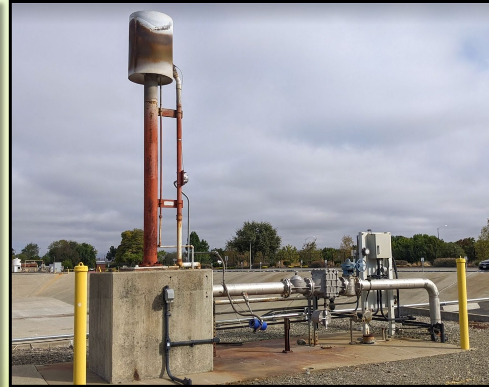
Biogas Flare Replacement
