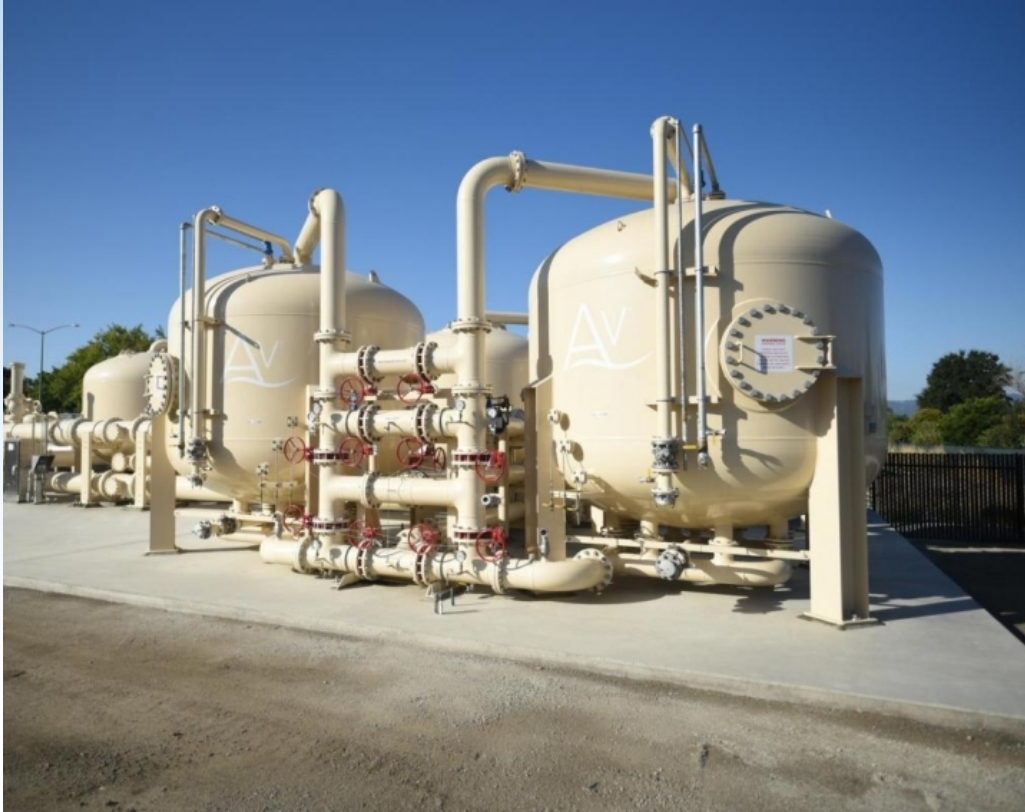
Stoneridge Well Ion Exchange Vessels.
