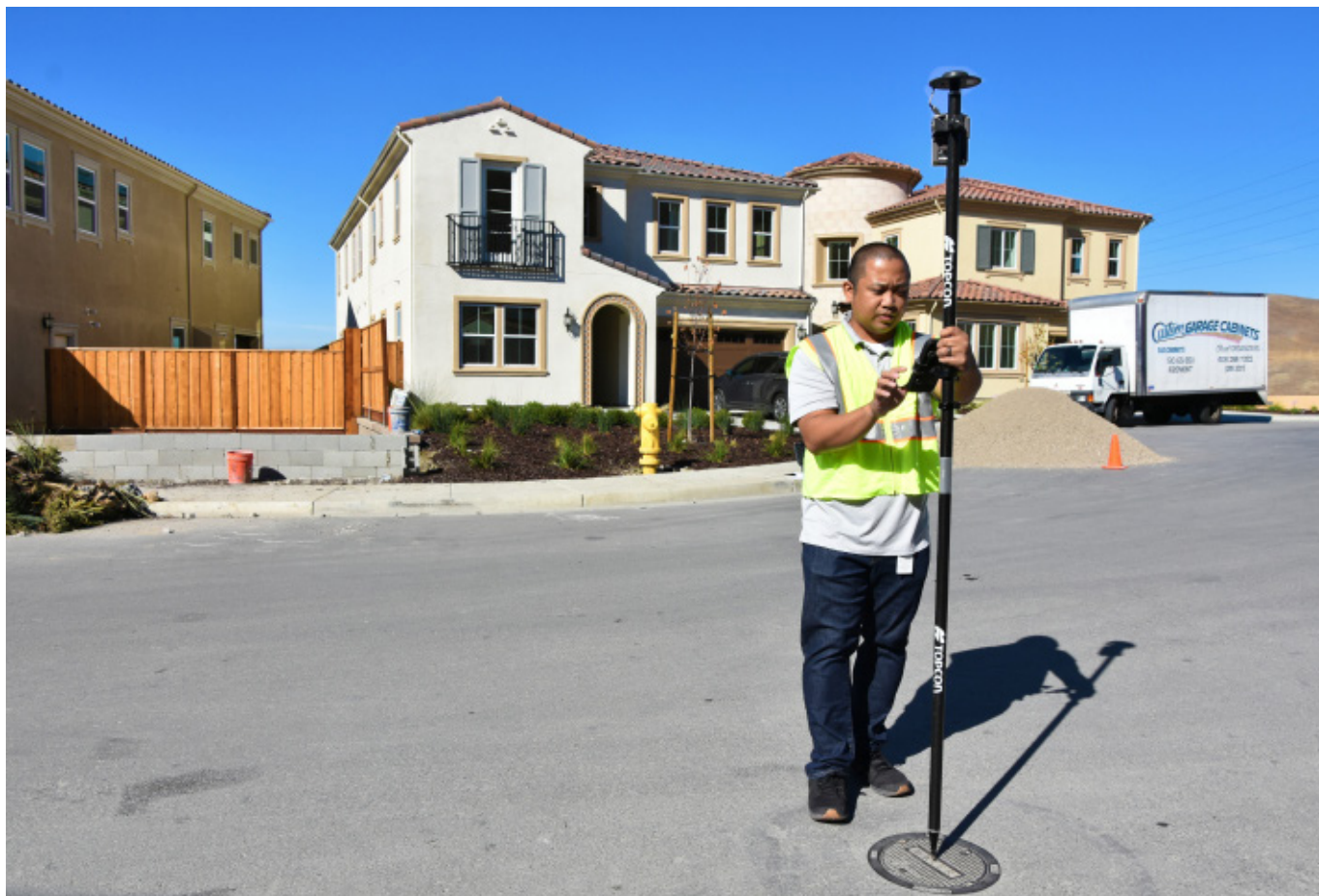
Engineering/GIS Technician Roper Macaraeg uses a locator to pinpoint a valve location in a new development that will be incorporated into the DSRSD's Geographic Information System. The new point will have valve information and service history to better track and maintain DSRSD's service area."
