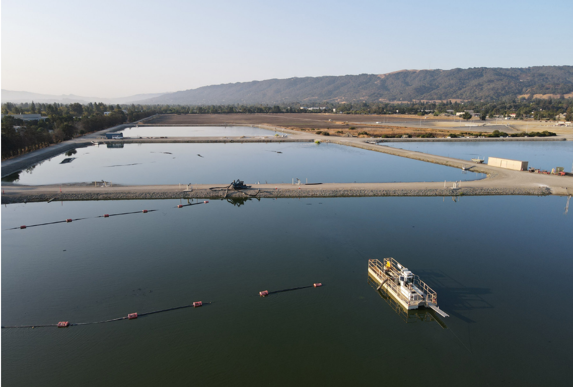
The dredge harvest biosolids from Facultative Sludge Lagoon Four.
