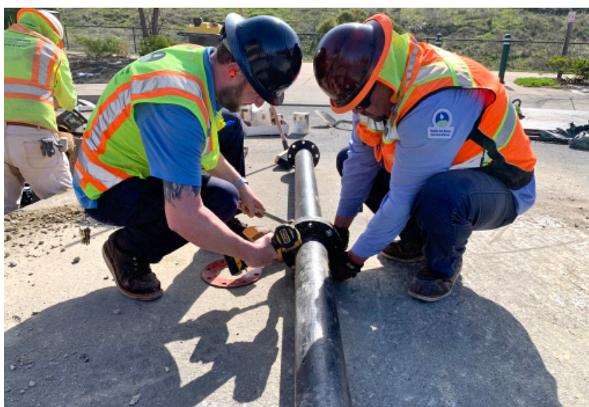
Senior Water/Wastewater Systems Operator Dan Pettinichio and Water/Wastewater Systems Operator II (On-Call) Eddie Gutierrez tighten nuts and bolts on a standpipe during an installation part of upgrading DSRSD's blow-off valves. Increasing the diameter from 2 inches to 4 inches allows operators to increase velocity when flushing water mains.
