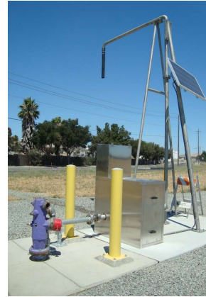
One of Central San's three hydrants (left) and a portable meter (middle) that contractors can use to obtain Central San's recycled water. Central San's Fill Station (right).
