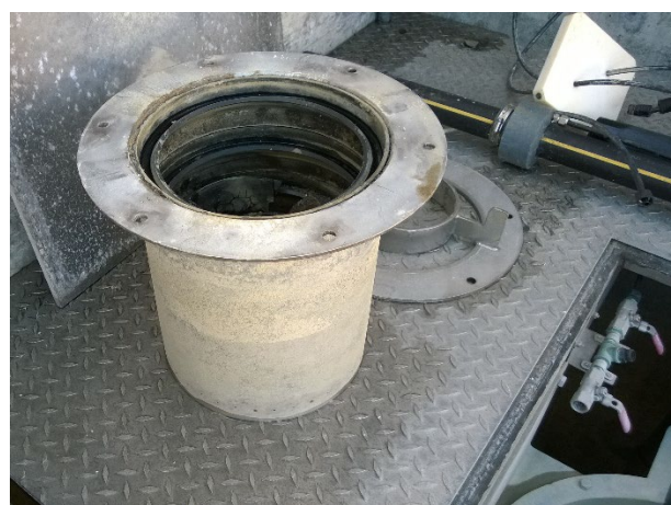
Photo: Broken cascade ring (left), sand filter wash zone assembly (right)
