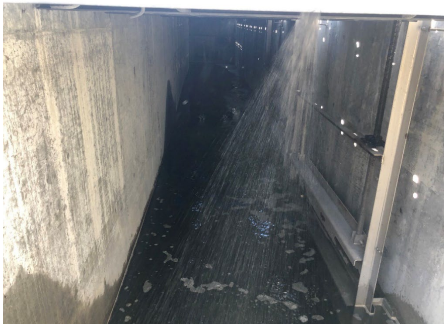
Photo: SFUV Channel 2 temporary spray system
