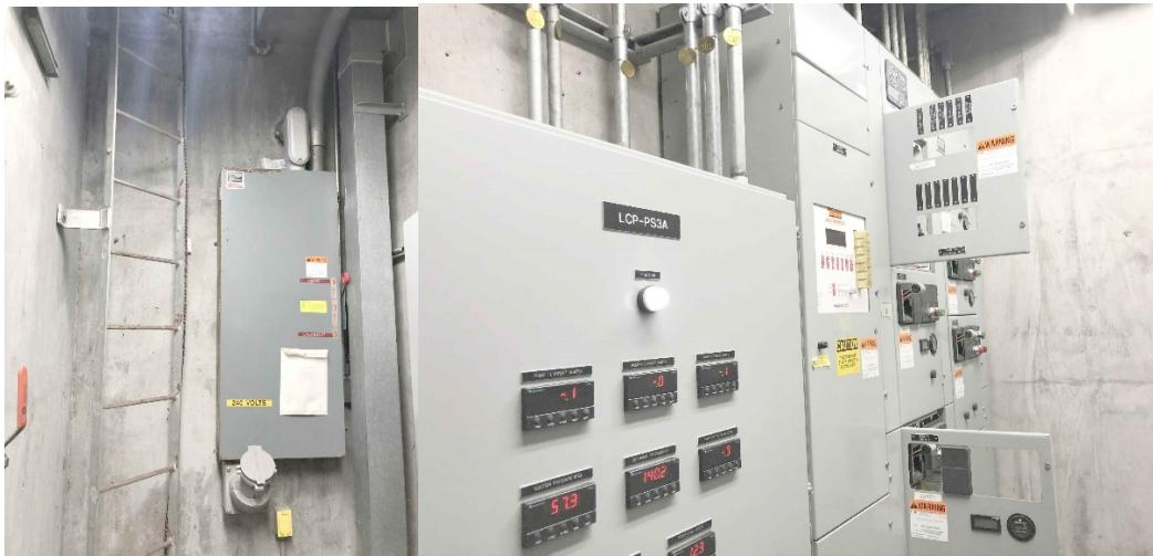
Figure 2: Existing Manual Transfer Switch Panel, Generator Receptacle, Lighting Control Panel, and MCC inside the vault
