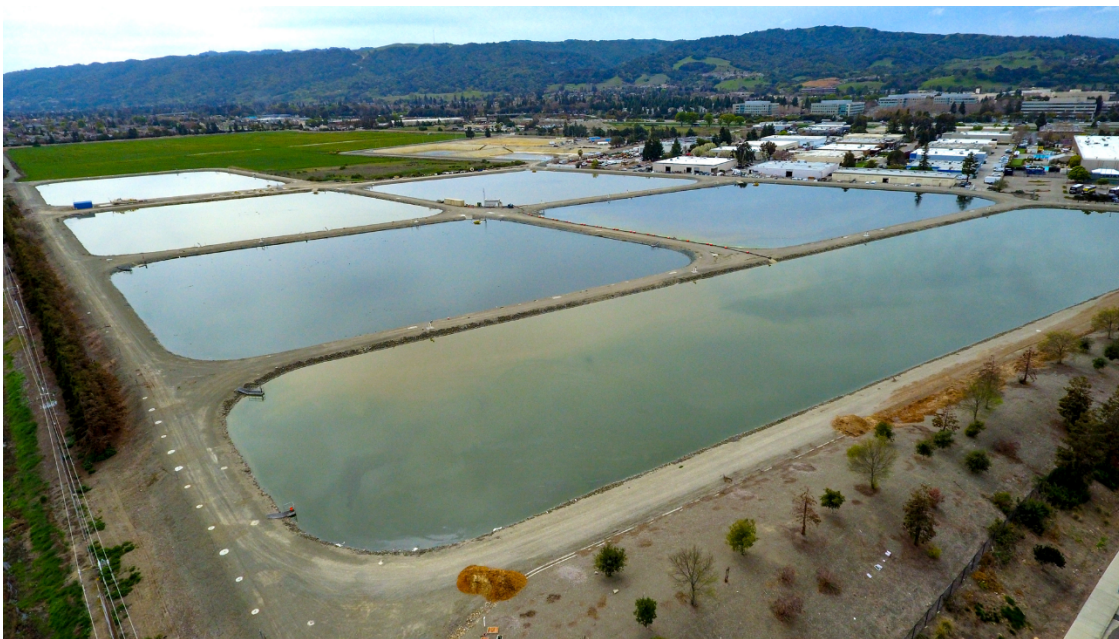
Figure 2 Facultative Sludge Lagoons
