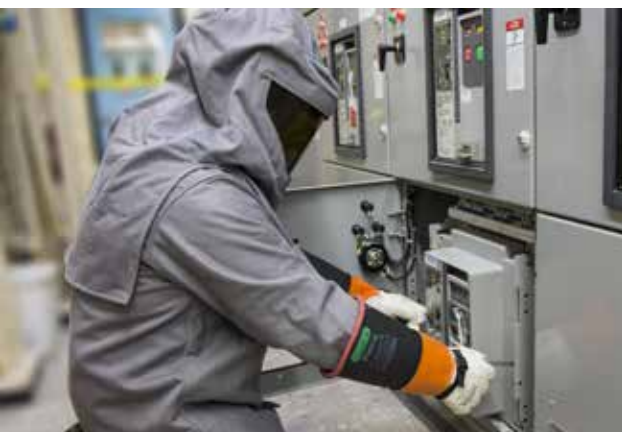
Electrician Il Brian Johnson installs a power distribution circuit breaker into an energized 480V distribution switchgear.
