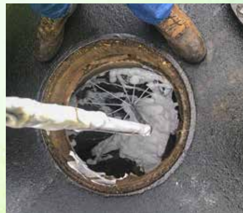
Foam is injected into the sewer line to clear pipes clogged by tree roots. The foam also prevents future root intrusion.
