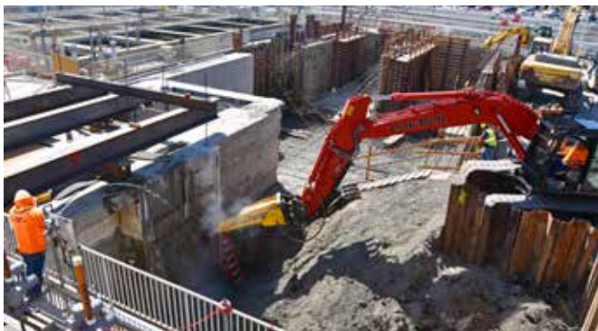
Primary sedimentation tank demolition and expansion.
