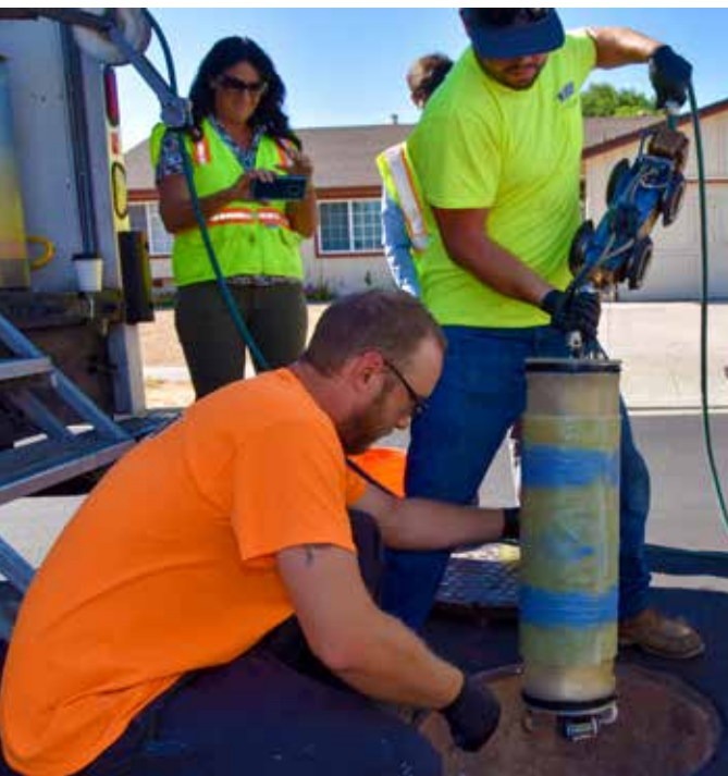
A contractor crew prepares to lower a sectional liner into the sewer for cured-in-place repairs in Dublin.
