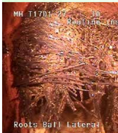
A closed-circuit video image shows a ball of tree roots blocking a sewer pipeline.
