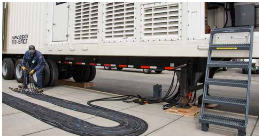
A contractor prepares the feeder cables for the emergency generator that temporarily powered the west end of the water recycling plant from mid-April to mid-June 2019.
