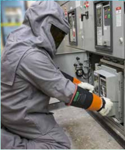
Electrician II Brian Johnson installs a power distribution circuit breaker into an energized 480V distribution switchgear.
