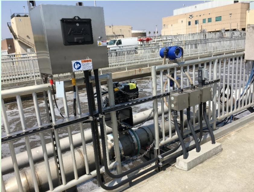
WWTP Aeration Basins Air Flow Control Valves
