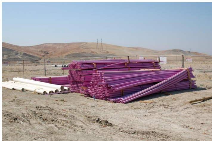
Developers install purple pipes for recycled water irrigation as new developments are built.
