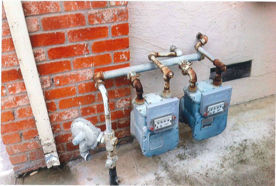
Doubled P.G.+E. meters for main house and Inlaw unit
