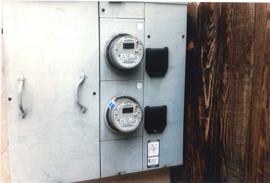
Doubled P.G.+E. meters for main house and Inlaw unit
