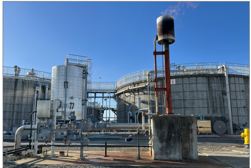
Figure 1: Existing biogas flare
