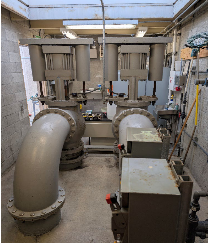
San Leandro Sample Station (Before) 2 Pressure Relief Valves
