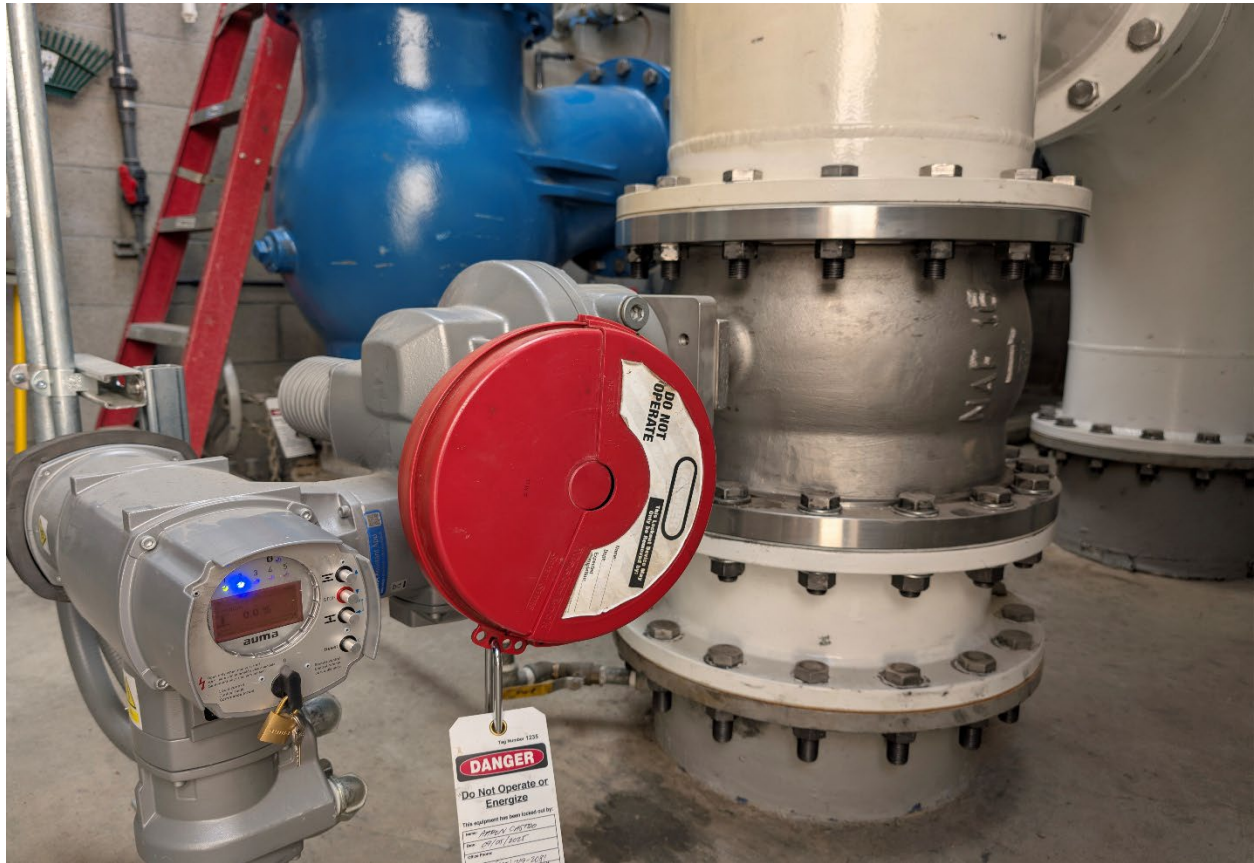
New Motor Control Valve
