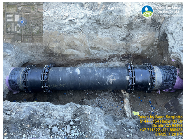
Photos: ( Left) Pipe break, (Right) Completed repair of 20-inch recycled water main using pipe provided by the City of Pleasanton.
