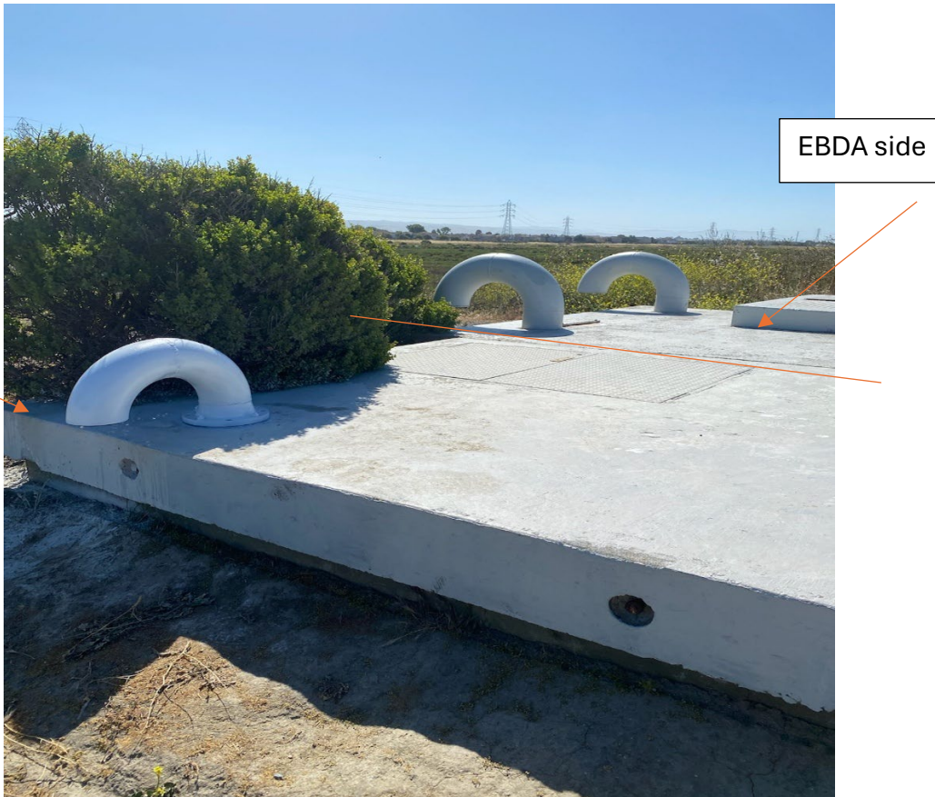
LAVWMA/EBDA Pipeline Connection Vault
